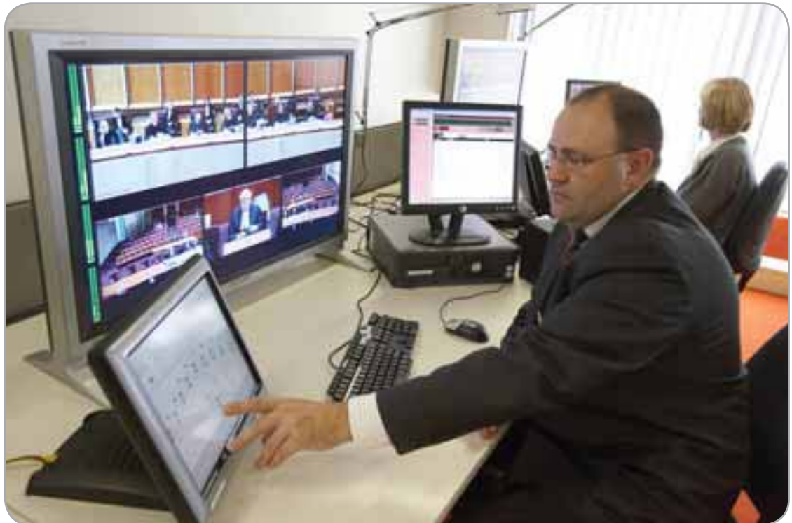
Video Switching Room.
