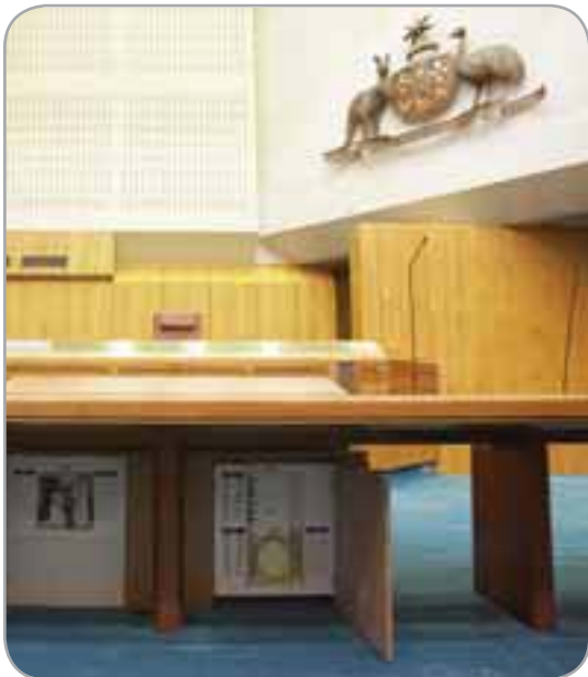
Control and Video Link Cupboard.
